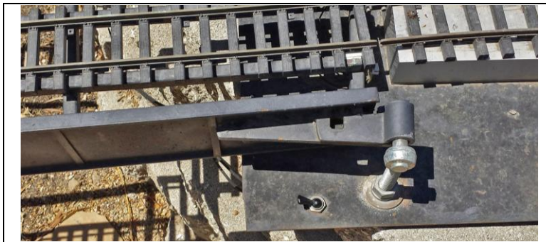
Outaluck Wye Switch Control
